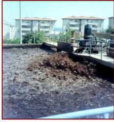
Mechanical (surface) aerators of activated sludge process treating wastewater
